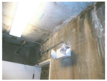
The photo (immediately above) shows an area at the east side of the Young building. The leaks here appear to be related to moisture entry at the patio between the two buildings. These leaks appear to be active and are likely to damage the doors and frame and the electrical lines and fixtures.
