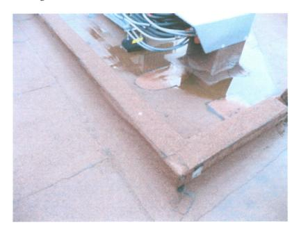
The photo (above) shows an example of several patches and short roofing caps that don't extend over the edges of the "parapets." It also shows one of the HVAC roof penetrations with messy use of foam sealant in place of a cap that would prevent water penetration.
