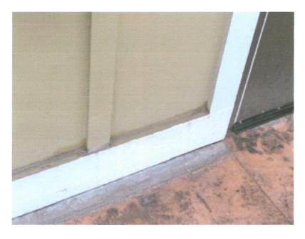
The photo (below) show some inconsistent and other defective trim and flashing practices. The photo on the right shows continuous flashing at the top of the "belly"
