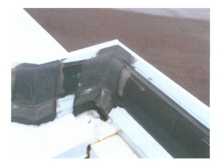
This photo (above) shows one of several areas at the expansion joint caps with one or two generations of repair. These caps are designed to cover airspaces between structural elements in the building. Leaks at such locations could travel several floors down and into the building and garage structure. The absence of roof venting systems could aggravate this problem.
