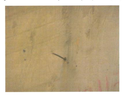
The photo above shows one of numerous form ties similar items that should have been trimmed during the finishing portions of the construction. There are also some areas with pieces of wood concrete-form material that have not been removed and areas of uneven concrete surfaces that should have been corrected.
